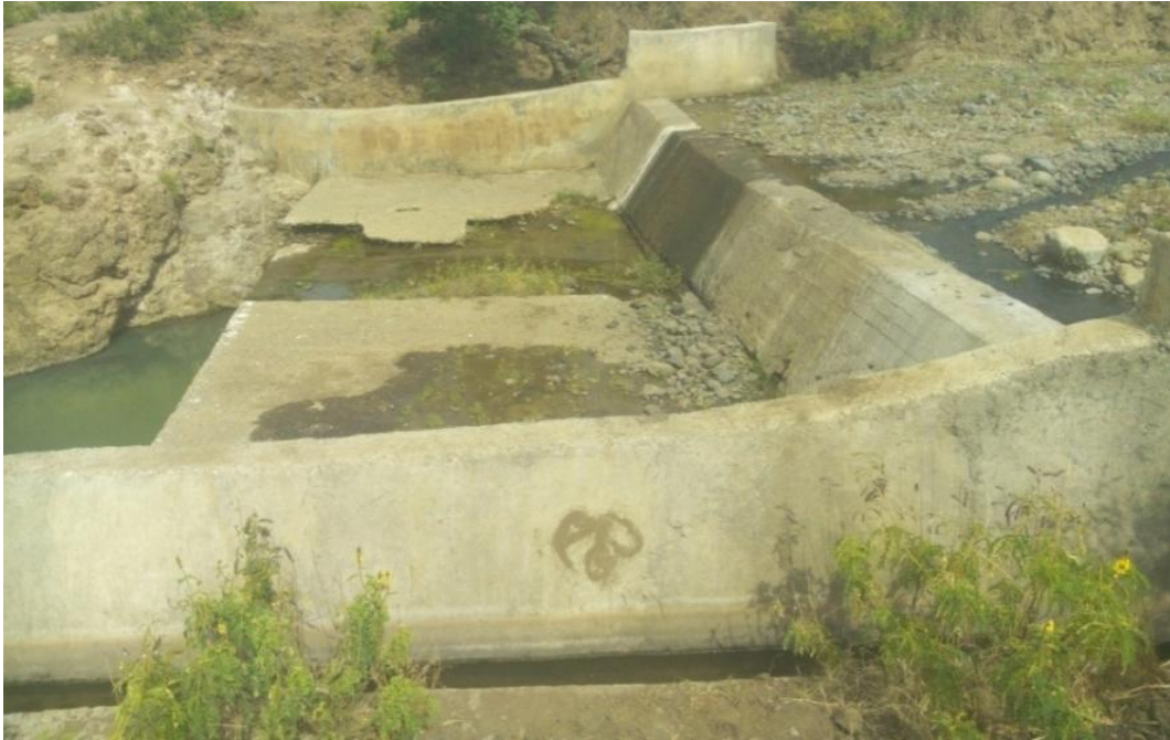
Figure 3. Scour at the downstream of the weir and abrasion of launching apron.
